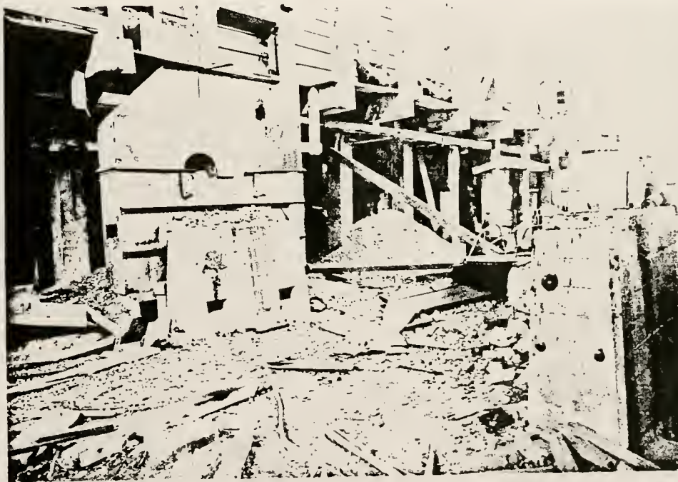
Figure 93. Revenue Mill (structure #34), concrete footings for ball mill, west view.
